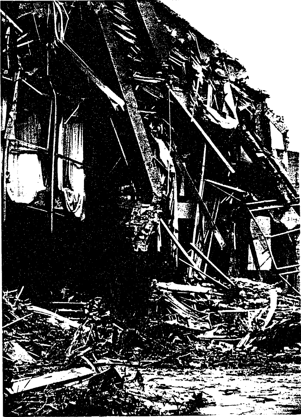
Figure 3. Collapsed reinforced-concrete structure after 1985 Mexico City earthquake
